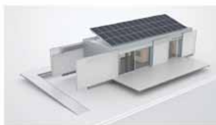
B. INITIAL OCCUPANCY: First modular unit for couple is set on site.
