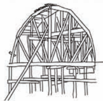
Wooden scaffolding was built during a 2 month dry period
